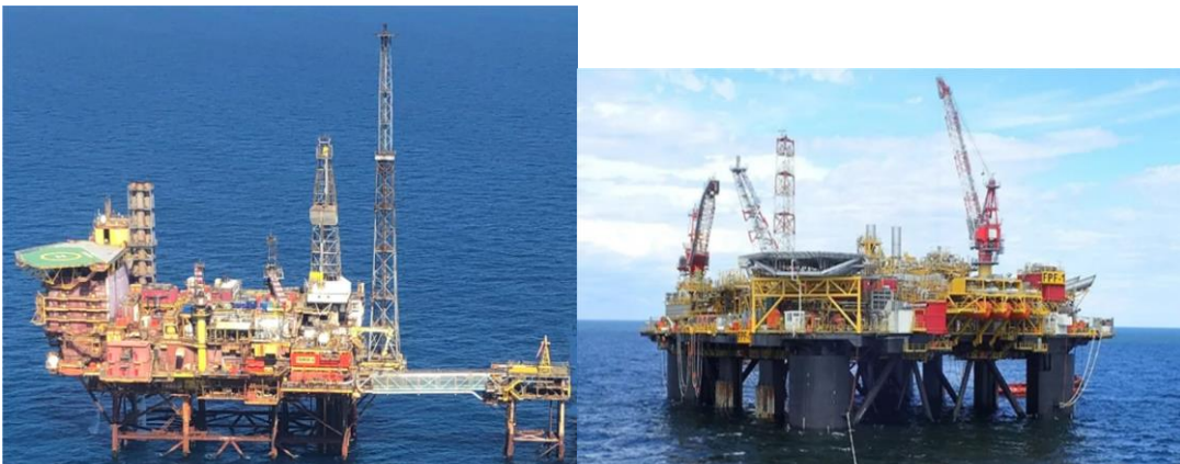
Figure 5 – Repsol Sinopec Fulmar & Ithaca FPF-1 platforms.
